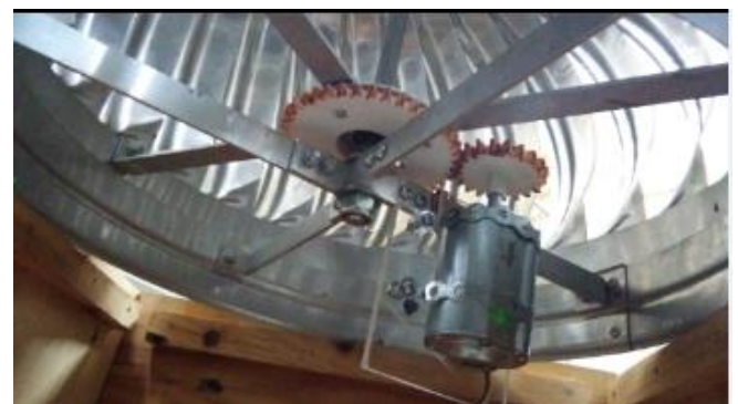
Fig.5. The installation of the gear
